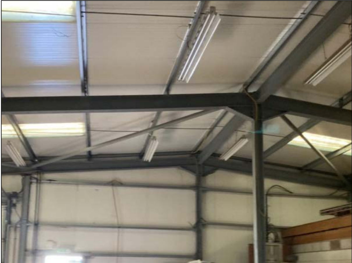
Photograph 13. Interior view of the storage building.
