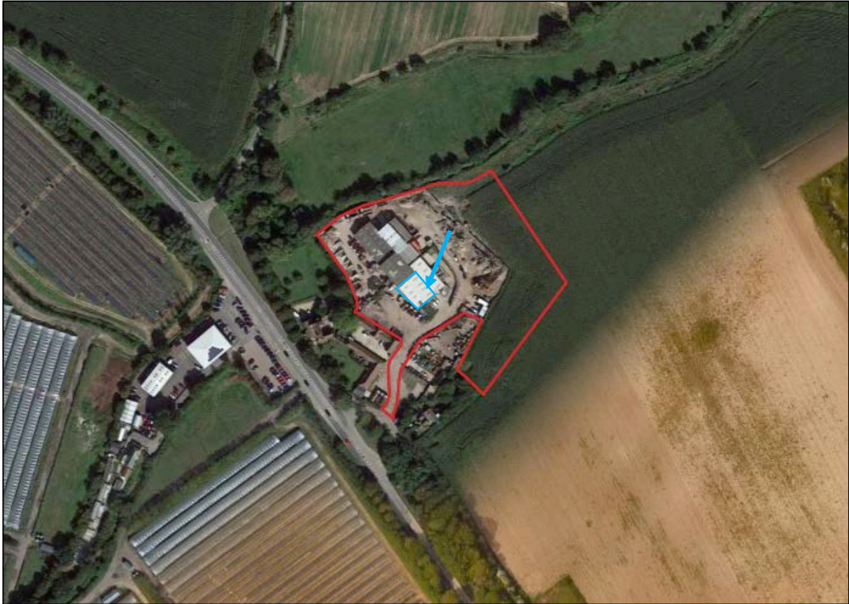
Figure 1. An aerial image showing the location of the site. The approximate site boundary is outlined in red and the storage building to be converted into new offices which was subject to a bat scoping assessment is shown with a blue arrow. Image produced courtesy of Google maps (map data ©2023 Google).
