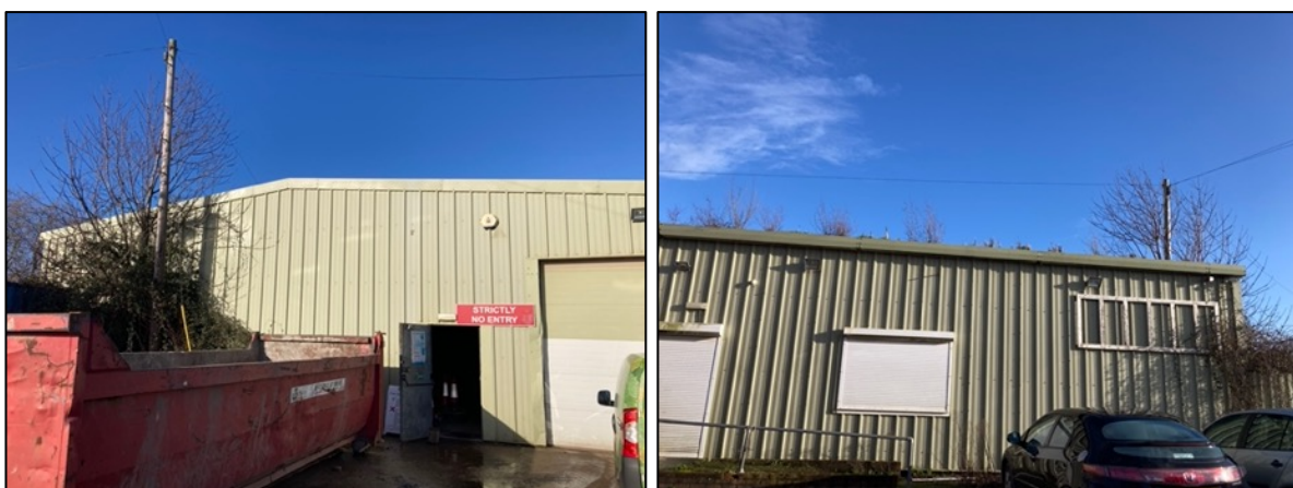
Photograph 12a (left) & b (right). Left - the southern elevation of the storage building. Right – The western elevation of the storage building.
