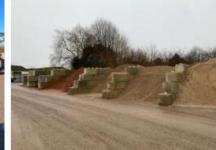
The aggregate storage bays are typically 3.2 metres high, 3.5 metres wide and 6 metres deep. The bays can easily to be moved or adjusted to reflect the site's operations.
