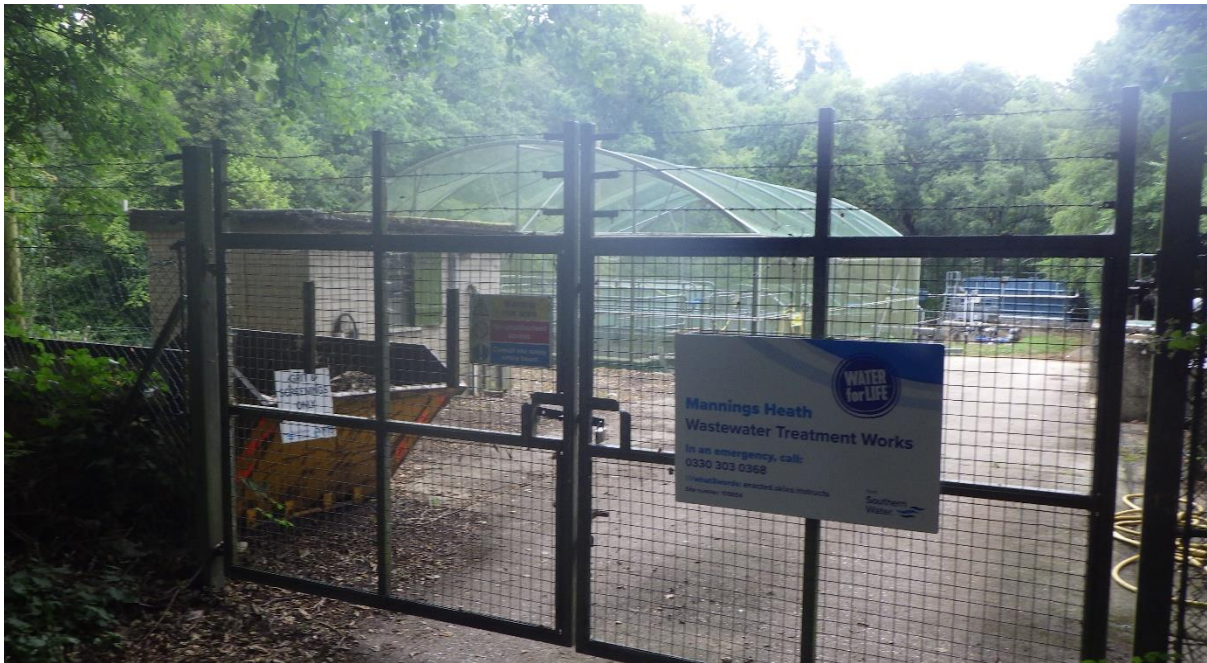
Plate 7.23: Mannings Heath Water Treatment Works at the eastern end of the pipeline scheme (looking north-west)
