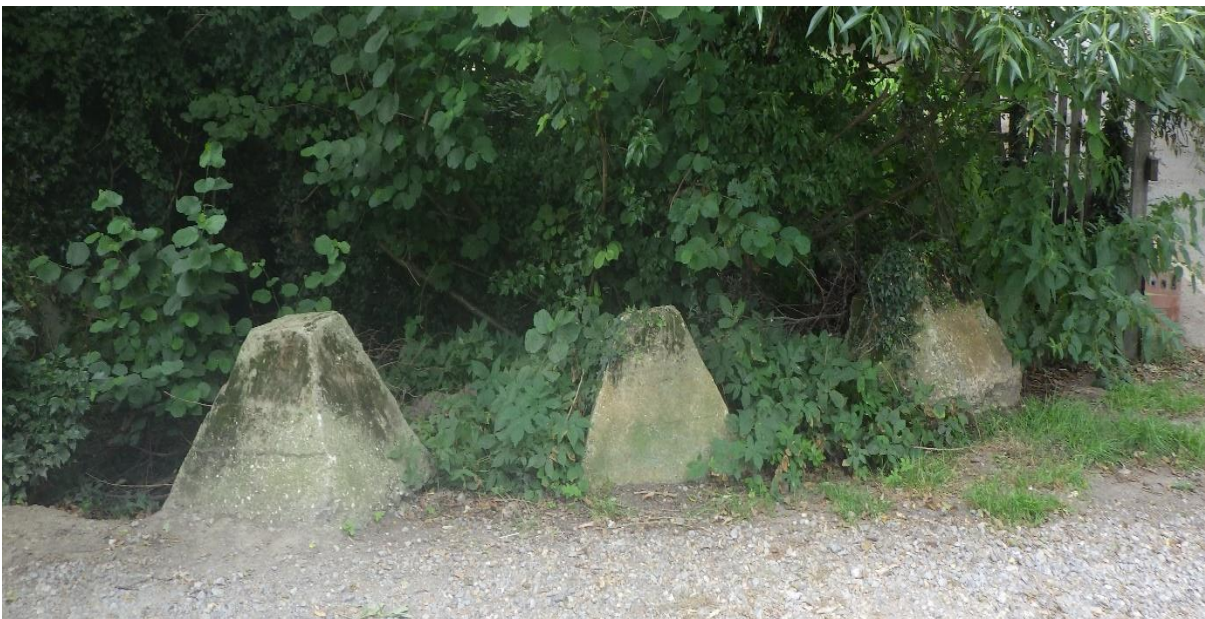
Plate 7.3: Anti-tank blocks (106) located by the stream at the entrance to Chesworth Farm along Chesworth Lane (looking east)
