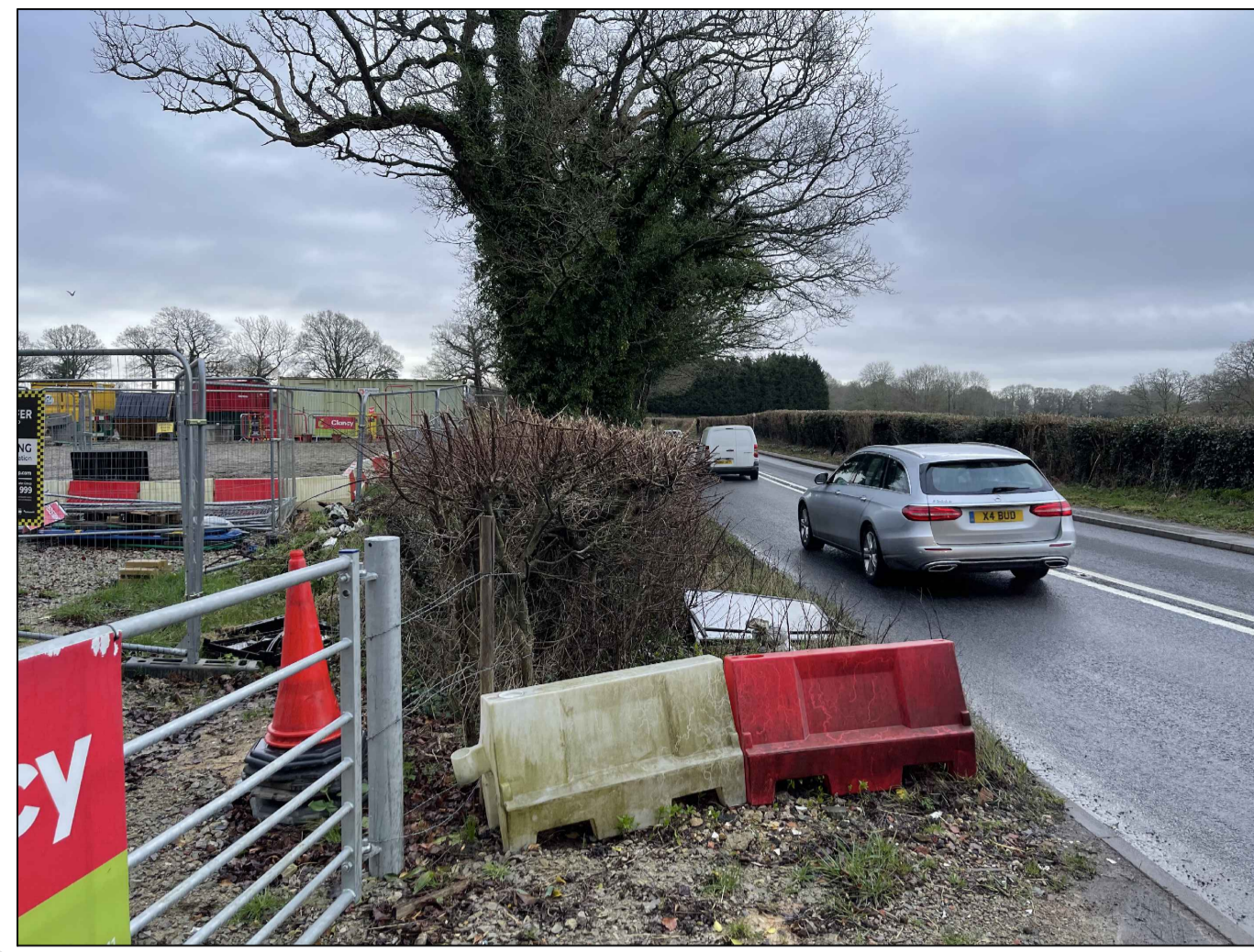
IMAGE 1 - VIEW FROM LEFT HAND SIDE OF ACCESS
