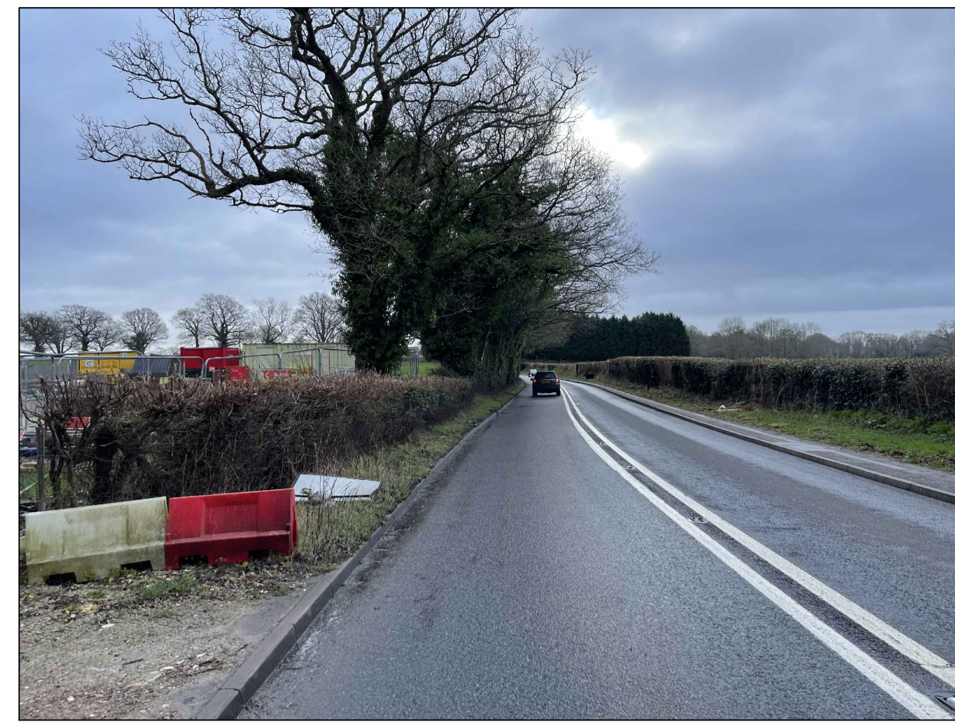
IMAGE 2 - VIEW FROM CENTER OF LEFT LANE
