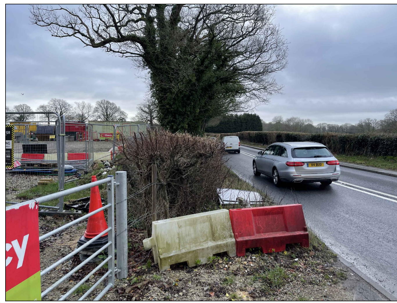
IMAGE 1 - VIEW FROM LEFT HAND SIDE OF ACCESS
